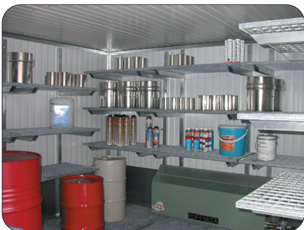
Equipped with shelving for use as small container store
